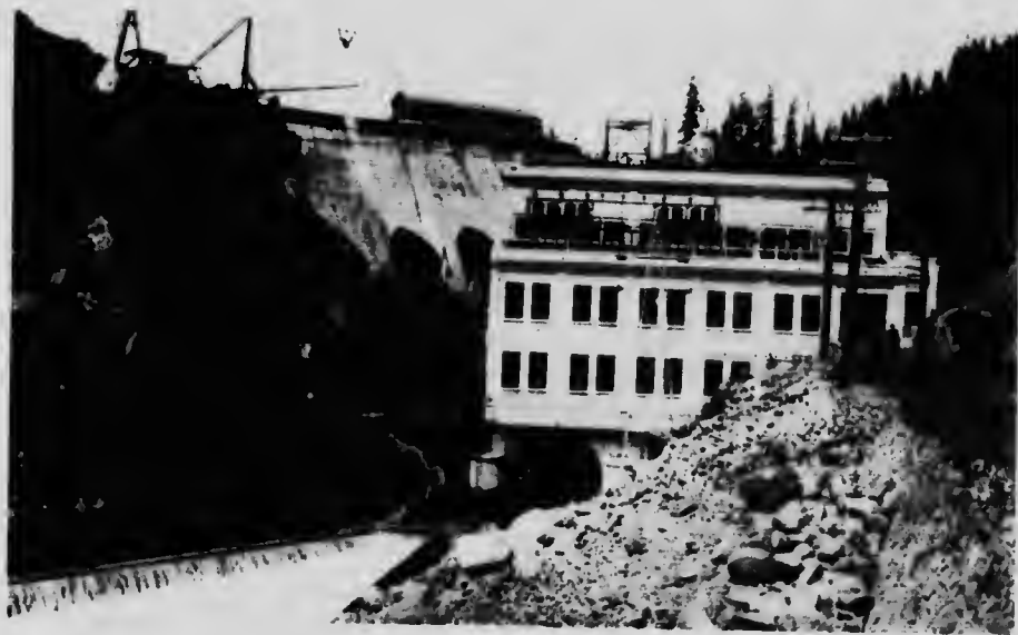
Stave Lake Development. Stave Falls Power House.
